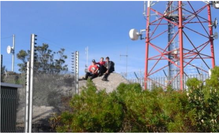
Witteklip (Lady's Slipper) repeater site
